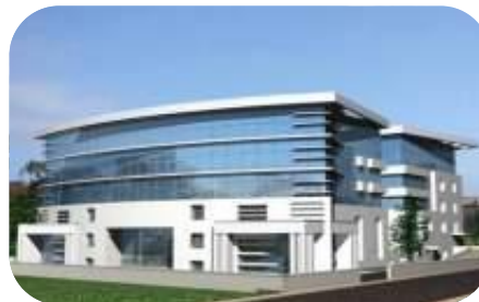
Engineering Centre and Bogie Technical Centre, Hyderabad
