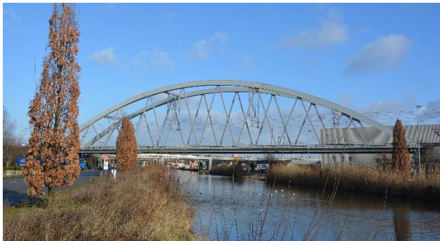
The KW51 railway bridge.
